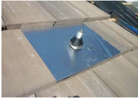
Figure 2a and 2b To meet one of the NRCA- and TRI-recommended methods of double flashing, the Quick Mount PV double-flashing kit consists of a primary peel-and-stick butyl flashing designed to interlay into the felt underlayment. A secondary preformed aluminum Flat Tile Mount flashing is applied at the top tile level.
