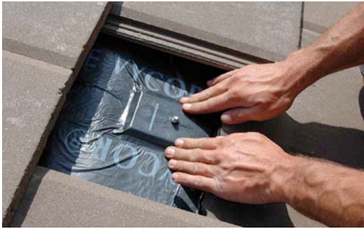
Figure 2a and 2b To meet one of the NRCA- and TRI-recommended methods of double flashing, the Quick Mount PV double-flashing kit consists of a primary peel-and-stick butyl flashing designed to interlay into the felt underlayment. A secondary preformed aluminum Flat Tile Mount flashing is applied at the top tile level.
