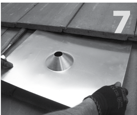
Cut a hole in the tile removed, with room to get the post through. Replace tile in position. Insert post and tighten into place. Install the 18"x 18" flashing and apply sealant around the opening.
