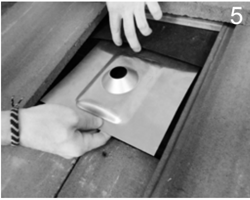
5 Place the Primary Flashing over the base plate, sliding the upper edge of the flashing under the course of felt paper above your base plate. If the next felt paper course is too high, you must place additional felt paper under its edge and over the Primary Flashing to continue the waterproof overlapping.
