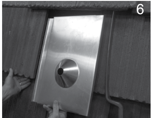
6 With the leading edge of tiles above still wedged up, lift left side tile and set aluminum flashing into place.
