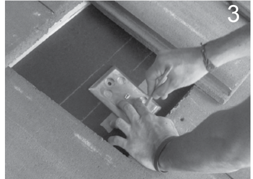
3 Use the base plate as a template to mark the drilling of the four attachment holes. Remove base plate, drill 11/64" pilot holes through the deck/block. Fill holes with sealant appropriate for the roof.
