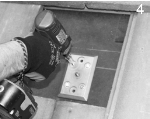
4 Insert grade 8 bolt under base plate in hex slot so threads point upward. Place base plate over pilot holes and secure with the four 1 1/2" lag bolts.
