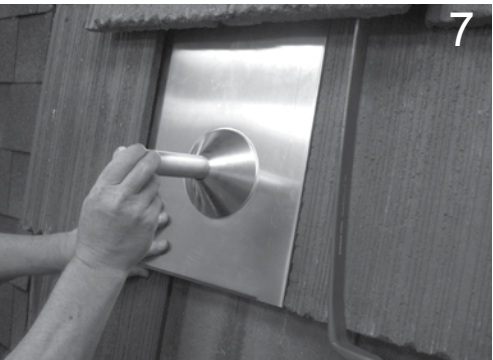
7 Insert post through flashing and secure to base on the Grade 8 bolt. Add sealant where post and flashing meet.
